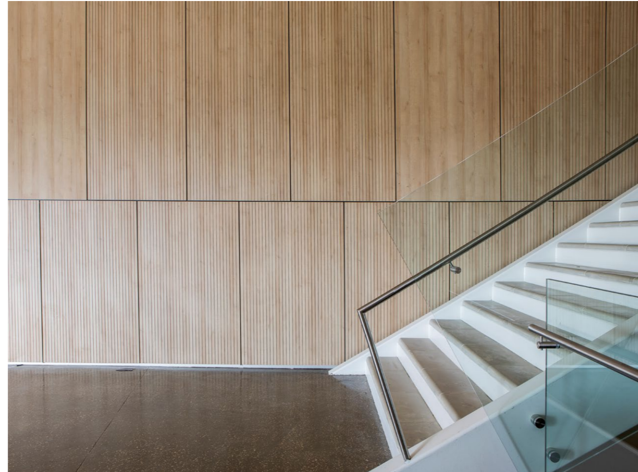
The project for the Nova School of Business and Economics campus in Carcavelos, Portugal, a reference building in Europe, incorporates several materials from the Innovus® decorative collection.
