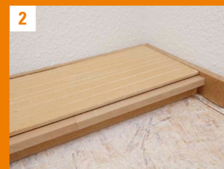
2 AGEPAN® TEP passgenau und fugendicht verlegen AGEPAN® TEP must be exactly laid with seamless joints
